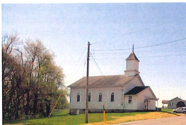
From Kellersburg Road – church west side
